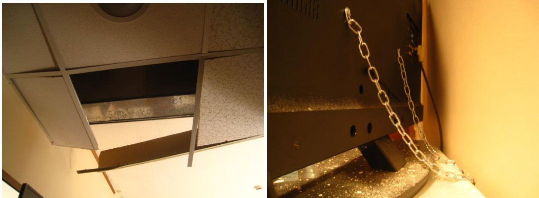
Left: example of non-structural damage. Right: Protective solution - prevent television from turning
