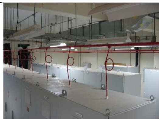
Cabinets tied together side by side using existing lifting hooks at top of cabinets
